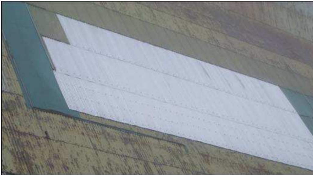
The final solution, using steel corrugated sheets. Cost £17,532:78p !
