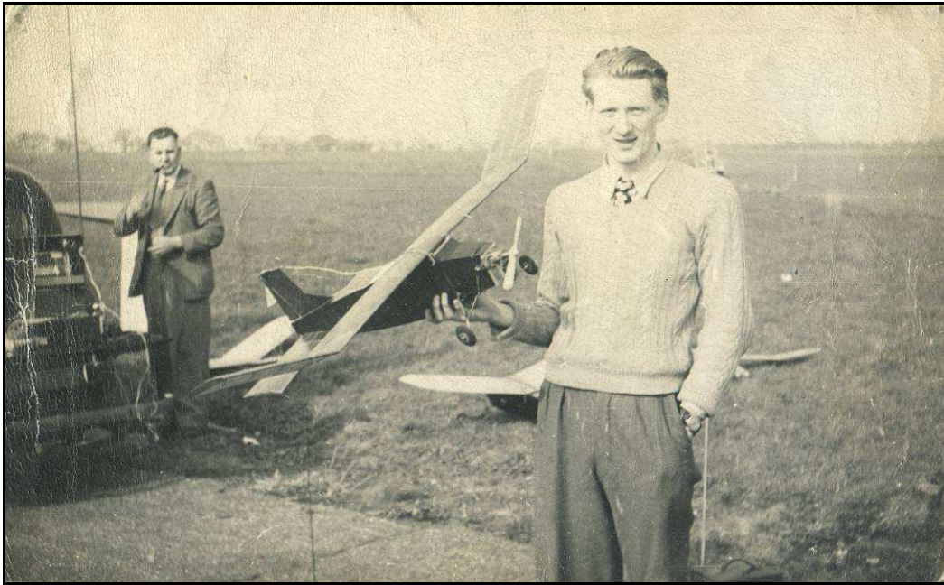
Here is a blast from the past, your editor with an R/C model in about 1953/4 The radio was a commercial ED set with the XFG1 soft valve Rx in a paxolin tube Ground based Tx with mico-switch pushbutton control Frog 100 powered with sequential rudder control by rubber powered actuator I lost it.
