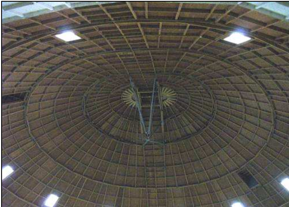
Interior view of the domed roof. Note: centre obstructions and bracing wires
